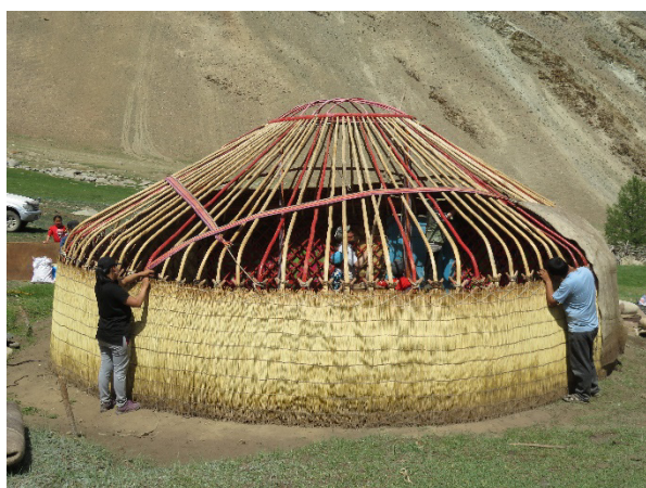
Photo 13 Tying the cords of wall felt
