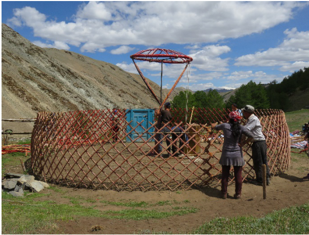
Photo 3 Crown wheel (шаңырақ) is erected using two poles (бақан)
