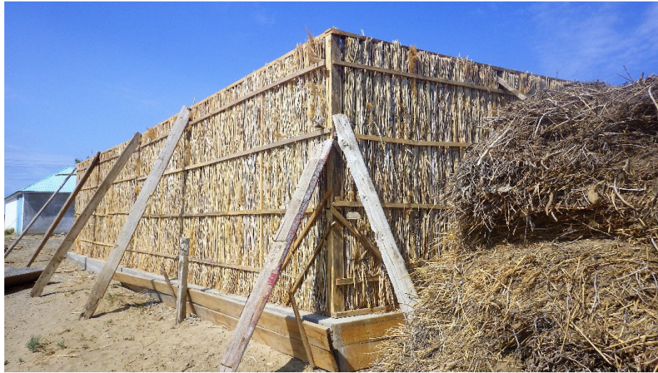
Photo 8. The livestock stall under construction without rooftop
