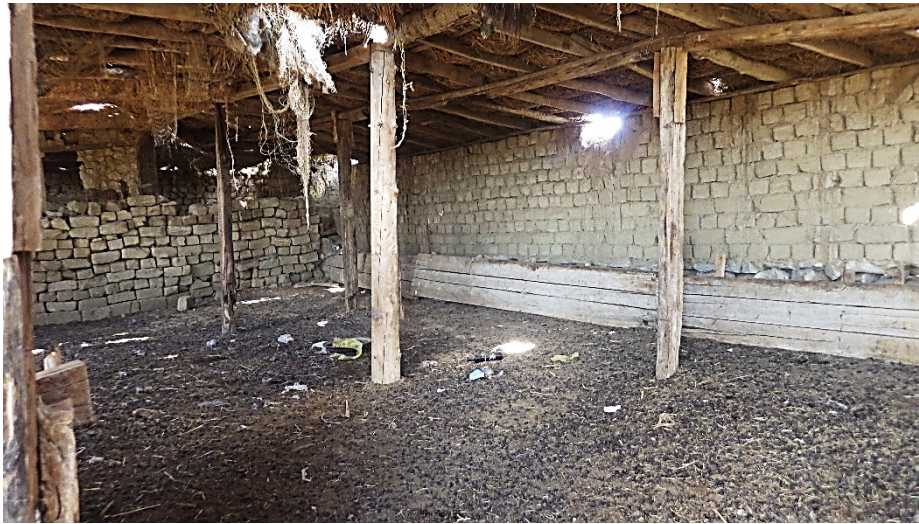
Photo 6. Livestock stall, constructed by woods and bricks
