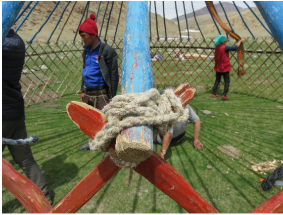
Photo 7 Roof poles tied to the walls by the rope (ұық бау)
