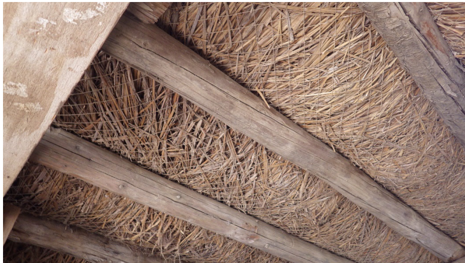
Photo 7. The roof with stretched fishing nets, wood, weeds and clays in the stall of Photo 6
