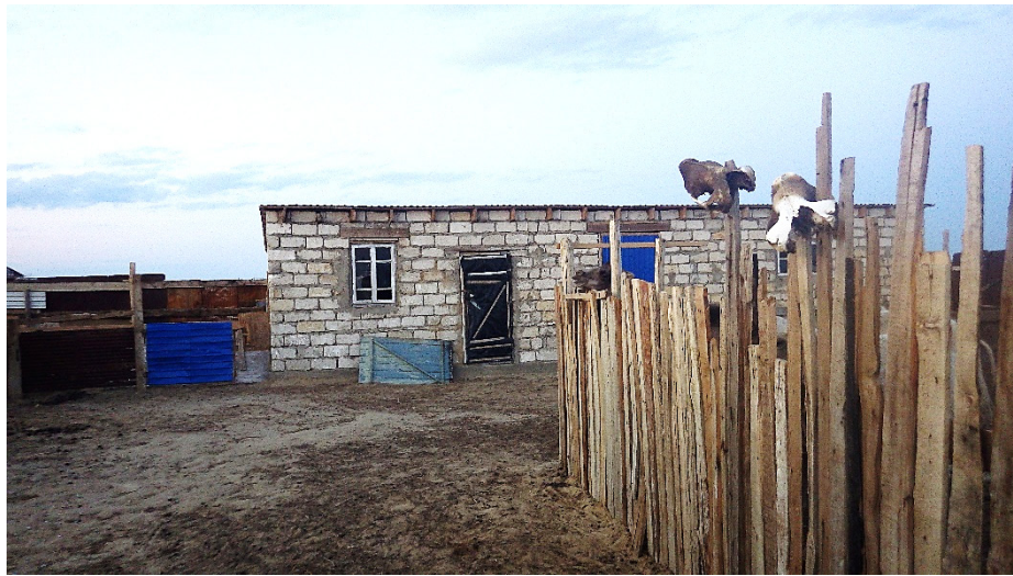
Photo 10. A modern but functionally deficient stall, using porous shell bricks
