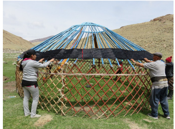
Photo 8 A wide belt-like cord (ішк арқані) is circled around the wall
