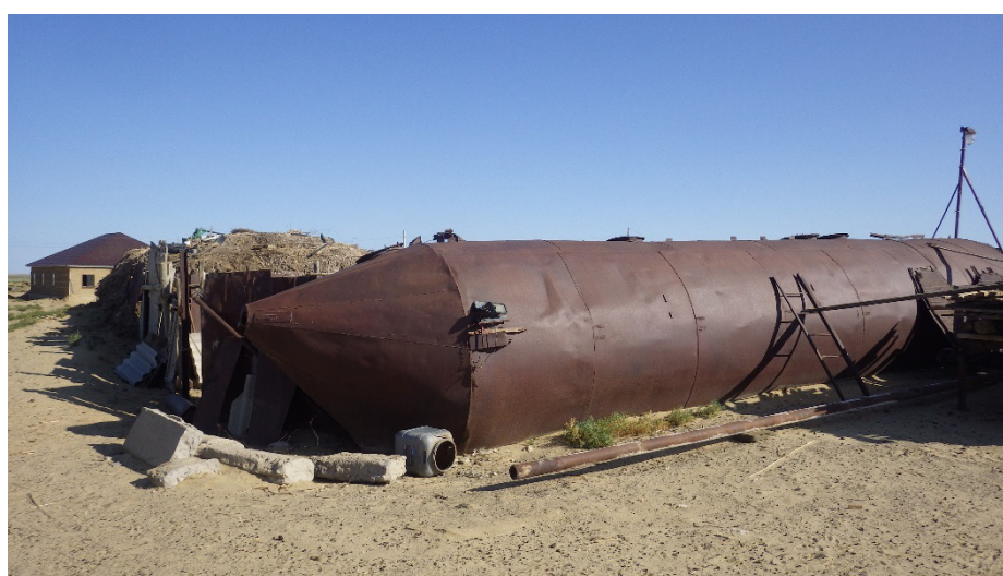
Photo 3. Metallic enclosure made of scrap iron from discarded ships
