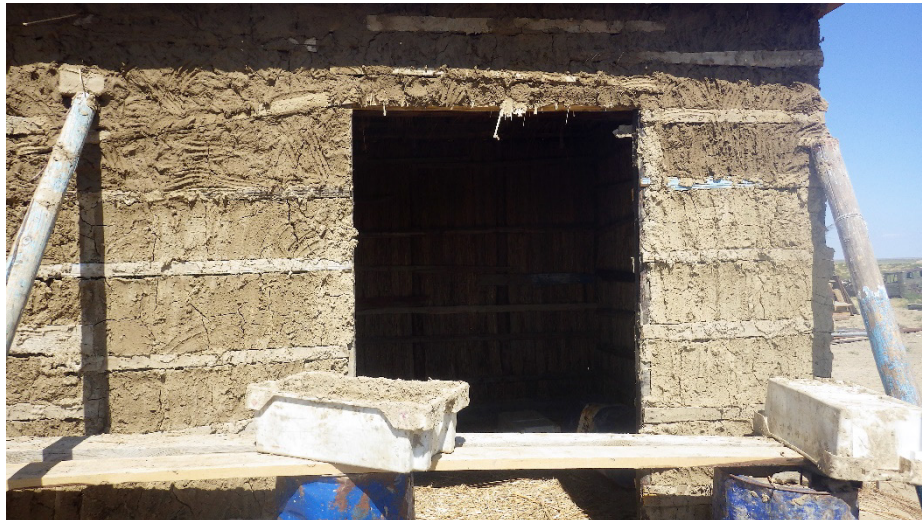
Photo 9. The high-quality and carefully structured livestock stall under construction
